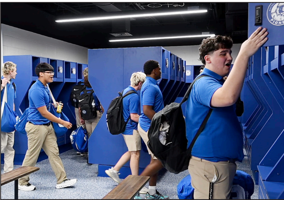
DHS students appreciate the complete renovation and upgrading of all five locker rooms on campus.
