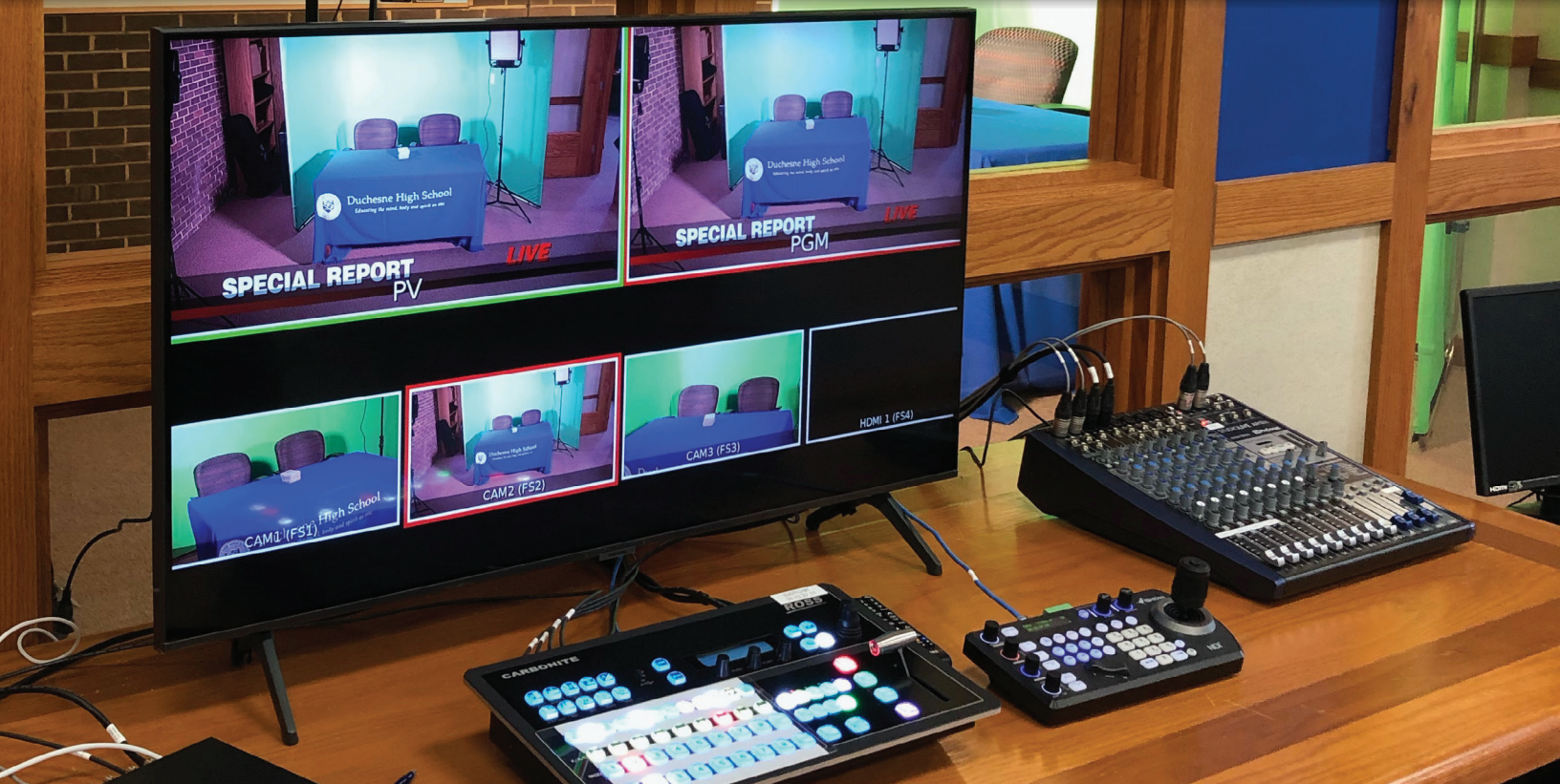
The switcher, camera controller, monitor, and audio board installed in Duchesne's new television studio as a part of 2022's Fund Our Future effort.
